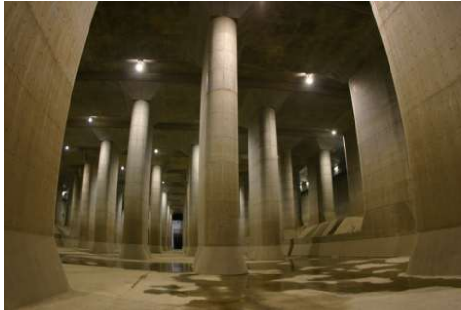
The “Surge Tank” of the Metropolitan Area Outer Underground Discharge Channel
